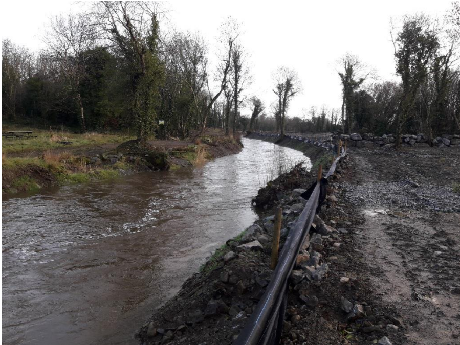
Figure 4; Regrading of Dunkellin complete
