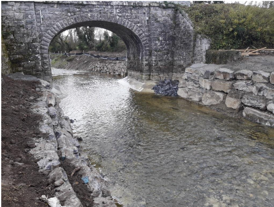
Figure 8; UB154 Railway Bridge
