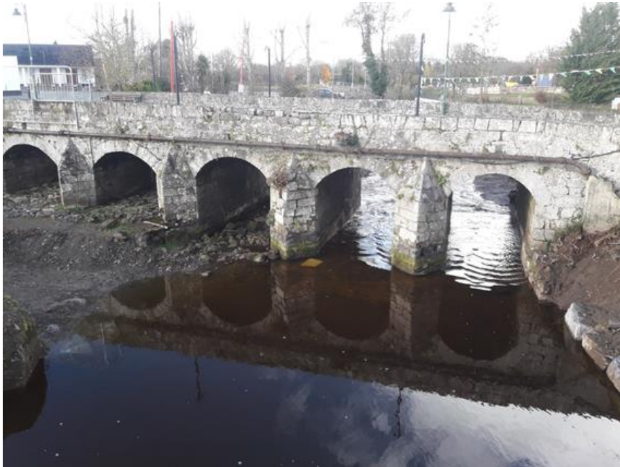
Figure 6; Regrading of Dunkellin complete
