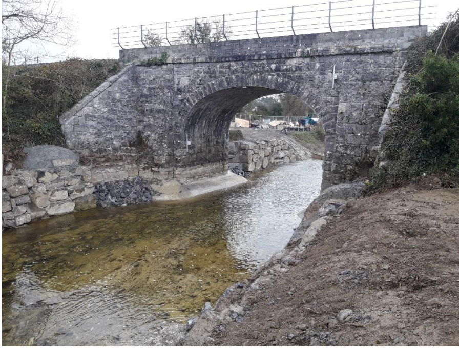
Figure 7; UB154 Railway Bridge
