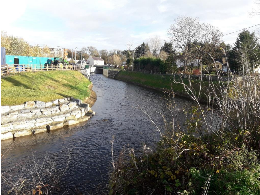
Figure 2; Downstream of Bypass Channel
