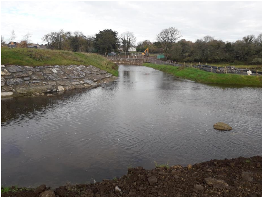
Figure 1; Upstream of Bypass Channel
