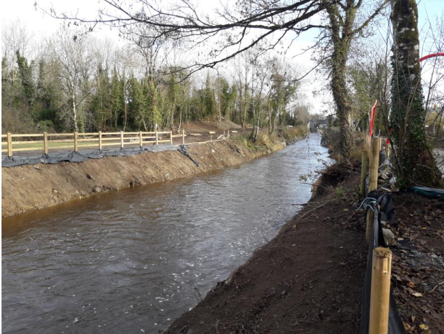
Figure 5; Regrading of Dunkellin complete
